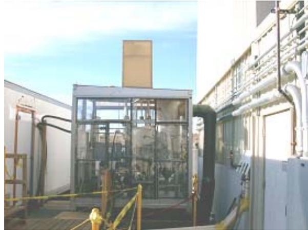
During 2001, AEA Technology completed design and functional testing of a directional nozzle system suitable for mobilizing and recovering sludge from the TA-50 facility Sludge and Influent Process Tanks prior to their return to service. During 2002, AEA Technology supplied a skid-mounted tank waste mobilization and retrieval system to the TA-50 facility at LANL to start mobilizing and retrieving the legacy waste from the tanks at this facility. Active operations commenced in October 2003.
