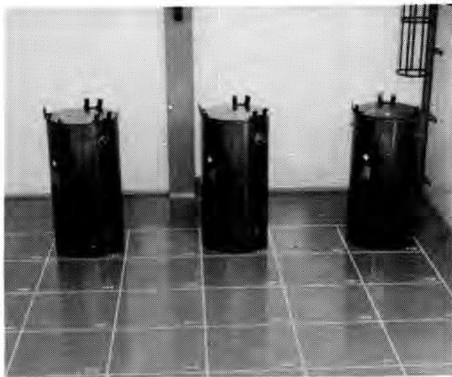
Fig. 4. CASTOR THTR/AVR in the storage hall.
