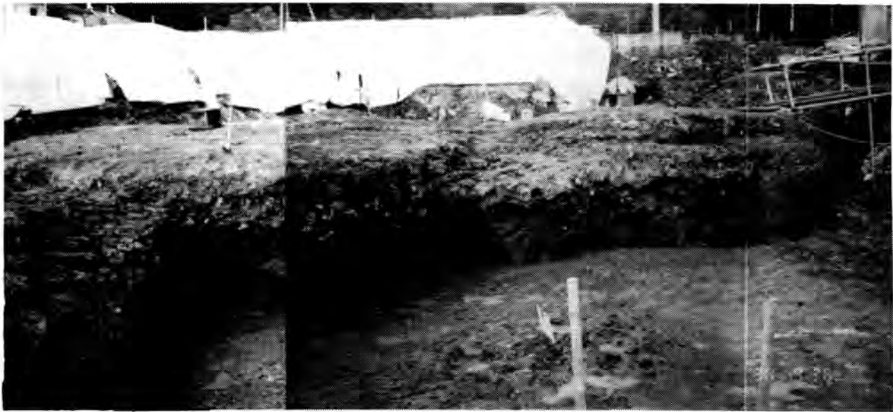
Fig. 5. Unearthed piles constructed in cohesive soil.
