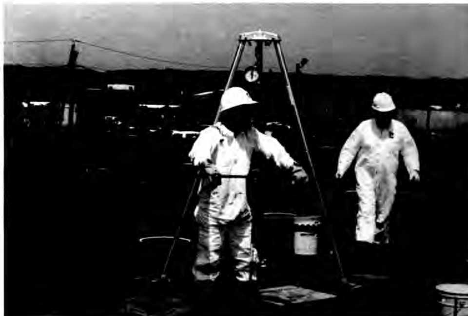
Fig. 12. Helical anchor field test in progress.
