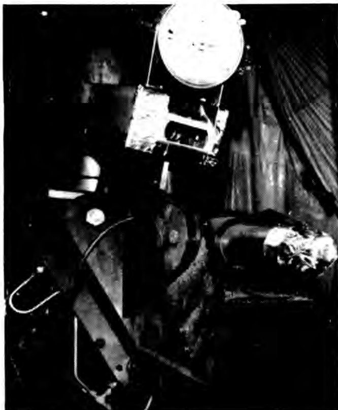
Fig. 3. Cutting torch assembly for vacuum vessel sectioning.
