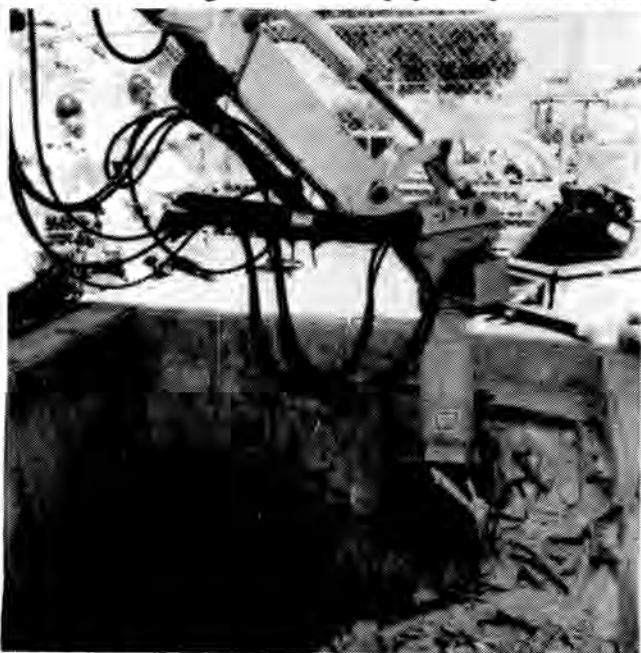
Fig. 6. Concrete removal equipment mock-up test
