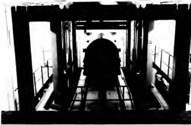
Fig. 3. Loading of the hoisting cage.
