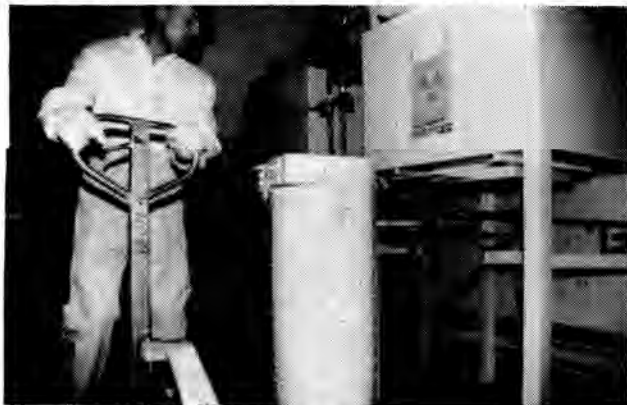
Fig. 5. Ion exchange column is changed from the IVO-CsTreat System's purification unit.
