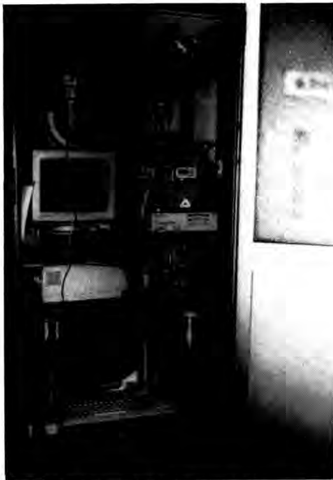
Fig. 6. Automatic sampling and measuring RI from off-gas.
