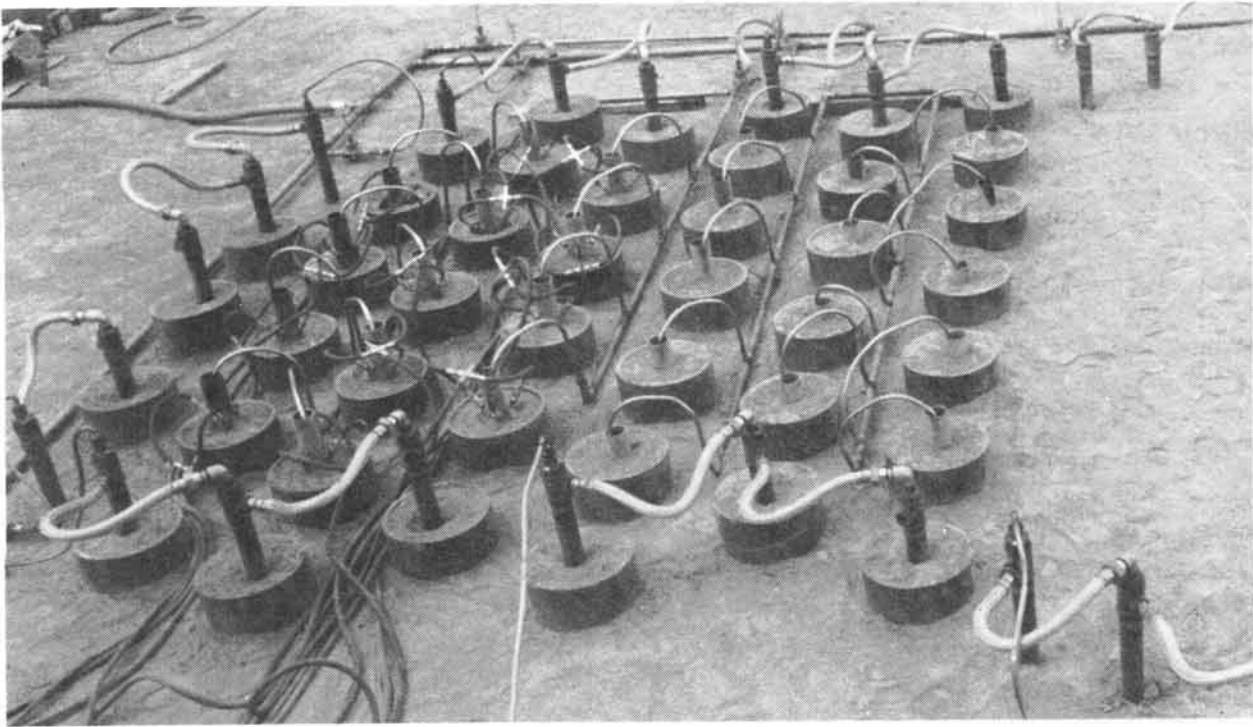
Fig. 1. Orientation of freeze pipes for several pits.
