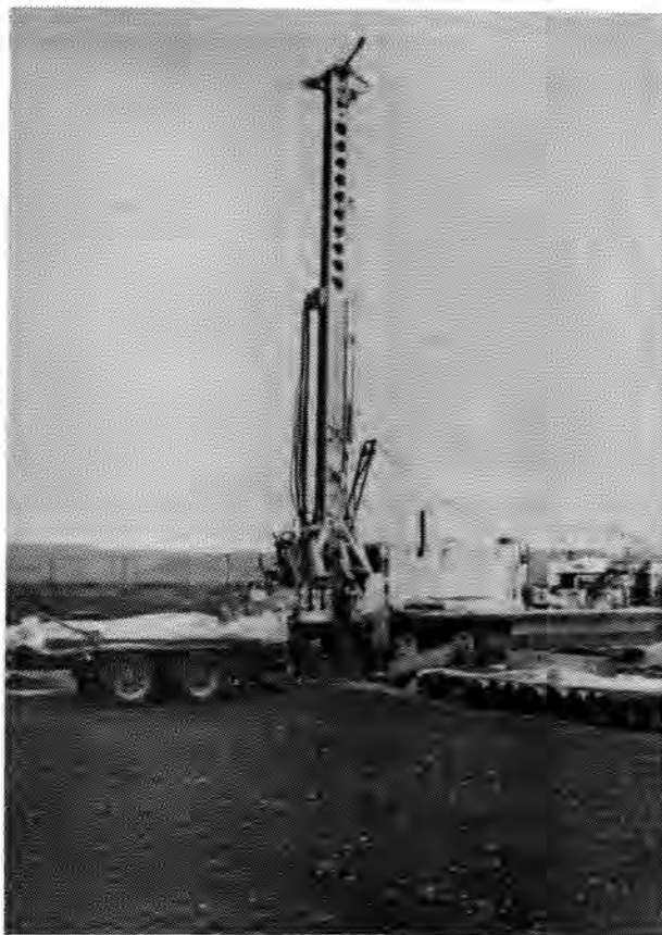
Fig. 4. Sonic drilling rig near the 216-Z-18 Crib.
