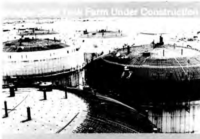
Fig. 2. Double-shell waste storage tanks under construction. Today, only the access ports are visible above the ground.
