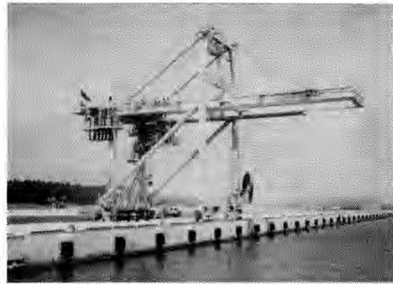
Fig. 6. 25 ton bridge type crane at Mutsu Ogawara Port.
