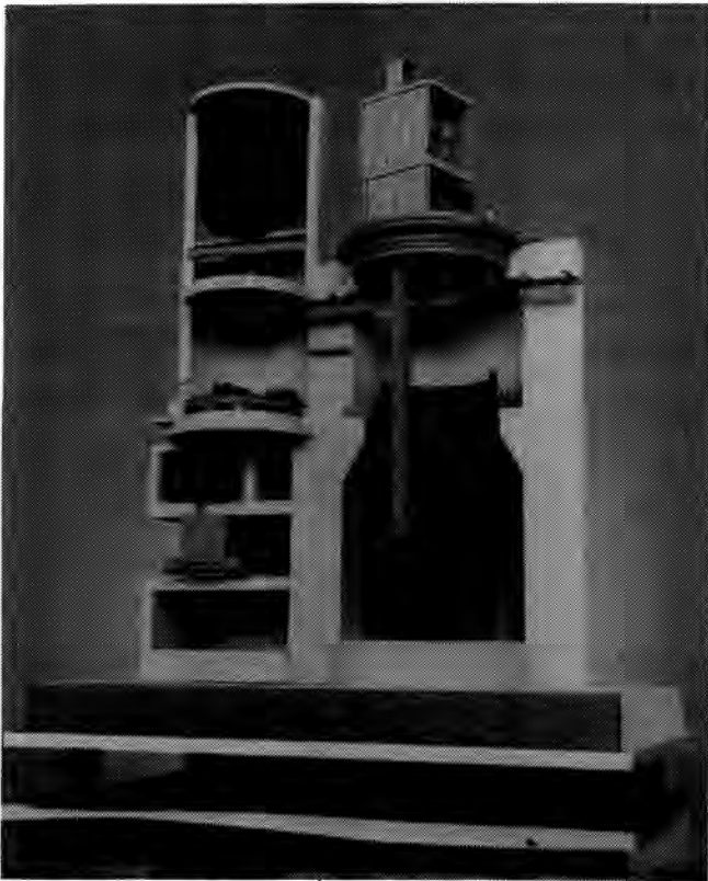
Fig. 3. Mock-up of WAGR dismantling machine.
