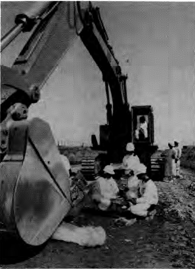
Fig. 3. Excavation and sampling of sediments during the 316-5 process trenches ERA.
