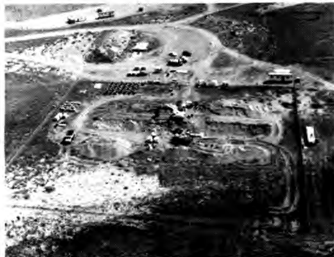
Fig. 5. Burial ground near completion of excavation.
