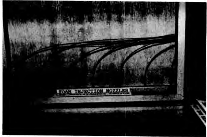
Fig. 7. Exit foam injection.
