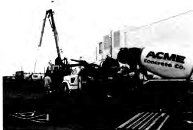
Fig. 3. Concrete Pump Used for Filling Burial Containers.
