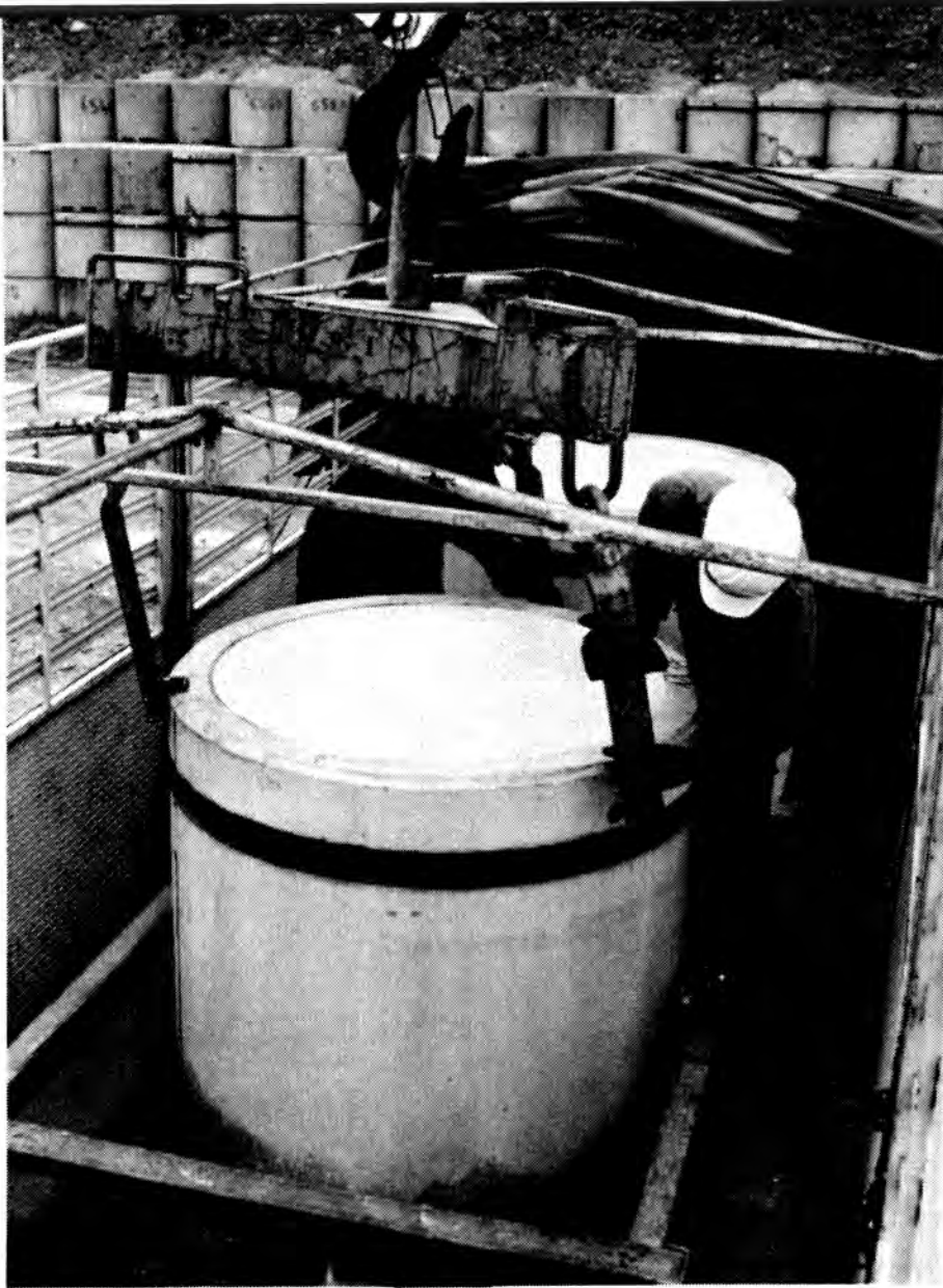
Fig. 2a. Filled Overpack Being Prepared for Transport to the Disposal Module at the Center de la Manche, France.
