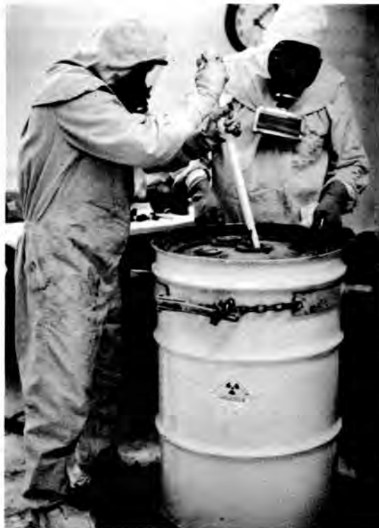
Fig. 1. Removal of a Probe Sample of Solidified Flyash.
