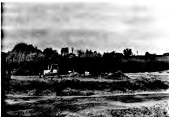
Fig. 9. Construction of Interim Storage Pile at MISS.
