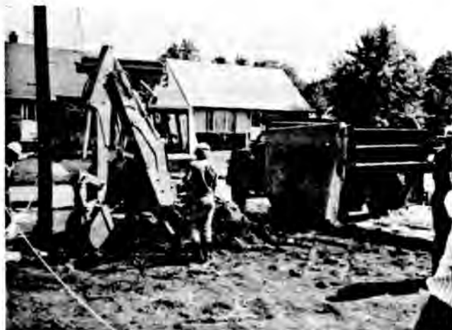
Fig. 10. Excavation at Maywood Residence.
