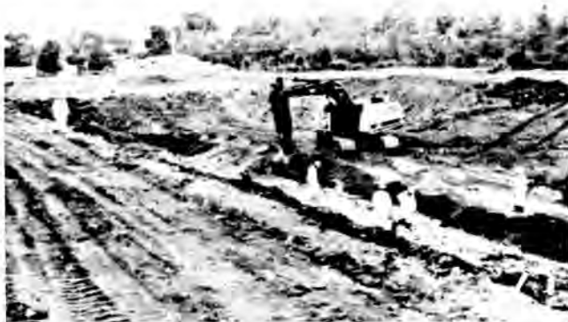
Fig. 4. Excavation of MML.
