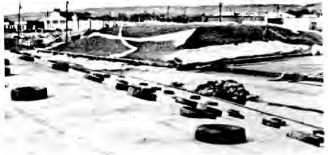
Fig. 3. Construction of Interim Storage Pile at MSP.
