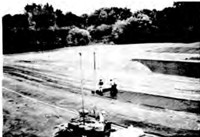
Fig. 6. Construction of Interim Storage Pile at WISS.
