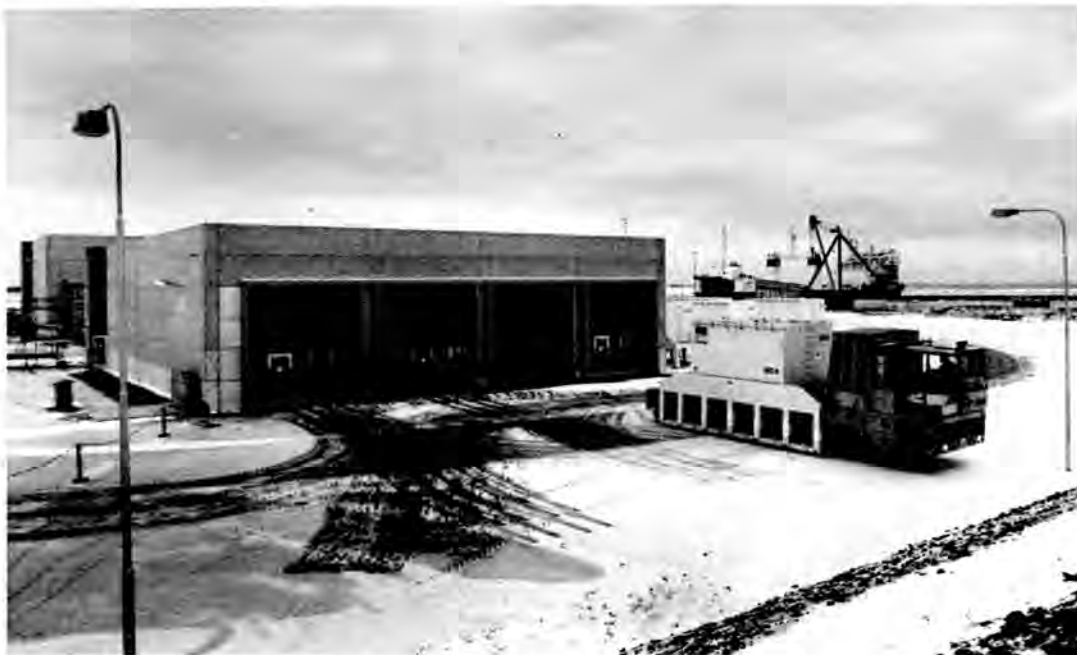
Fig. 4. Unloading of Transport Containers From M/S Sigyn to the Terminal Building at SFR.
