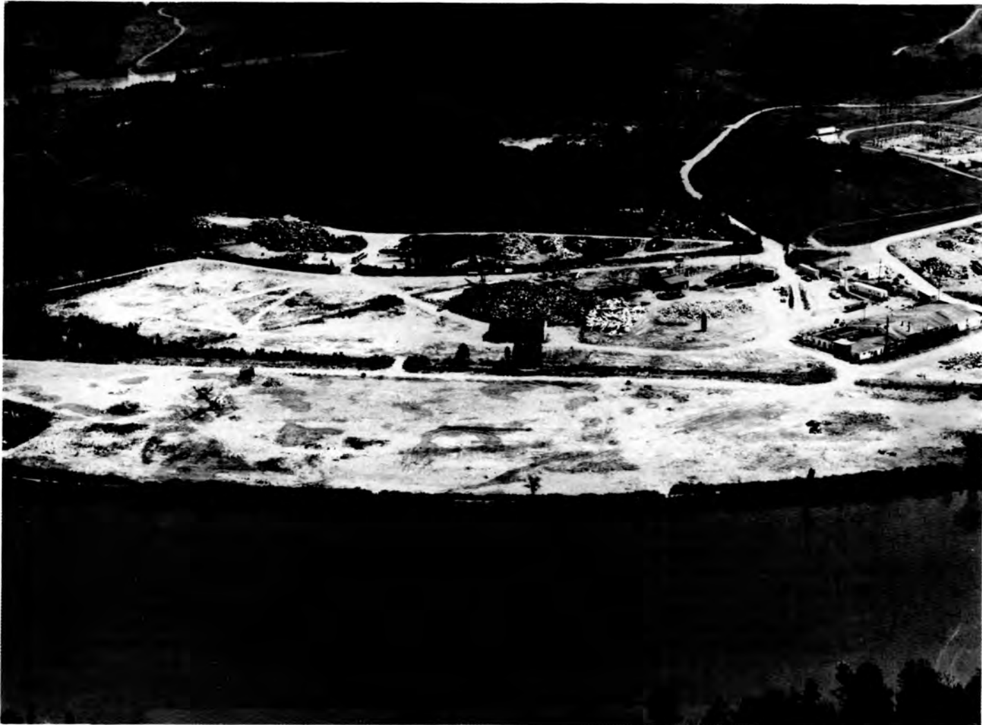
Fig. 7. Aerial View of Scrapyard After Cleanup - August 1985.
