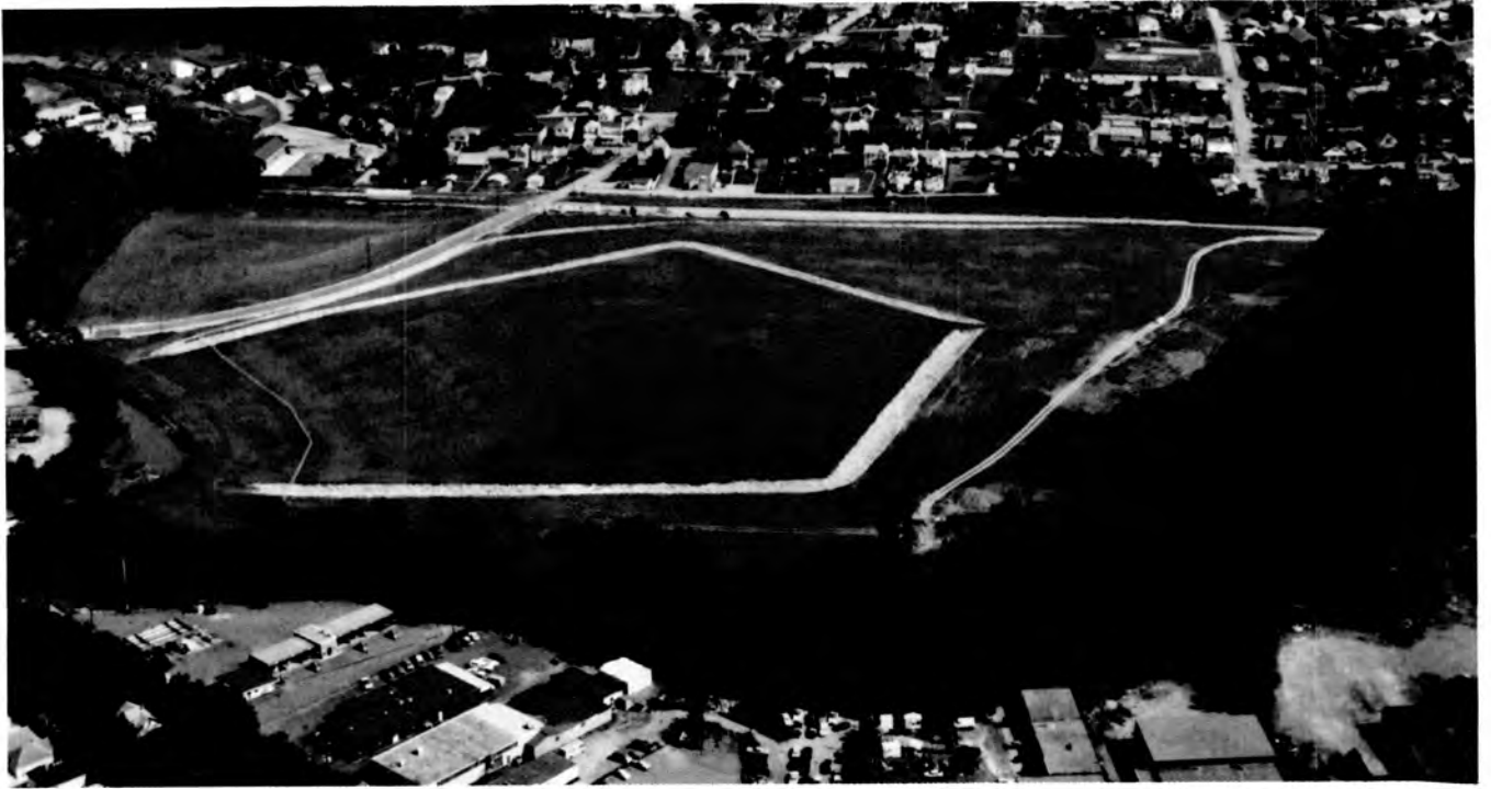
Fig. 1. Completed Tailings Deposit at Canonsburg, PA
