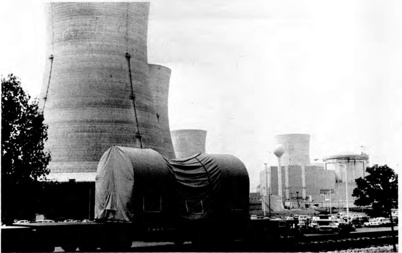
Fig. 5. Rail Cask and Railcar Ready for Transport at TMI.
