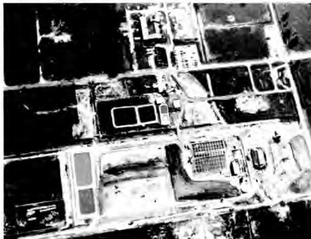
Fig. 4. Aerial View of the NFSS Waste Containment Area Showing the Partially Completed Interim Cap and Building 411.
