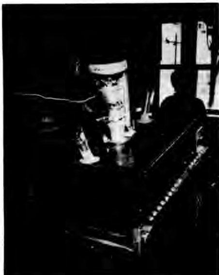
Fig. 1. The CUA/VSL Mini-Melter Tilted for Glass Pouring.
