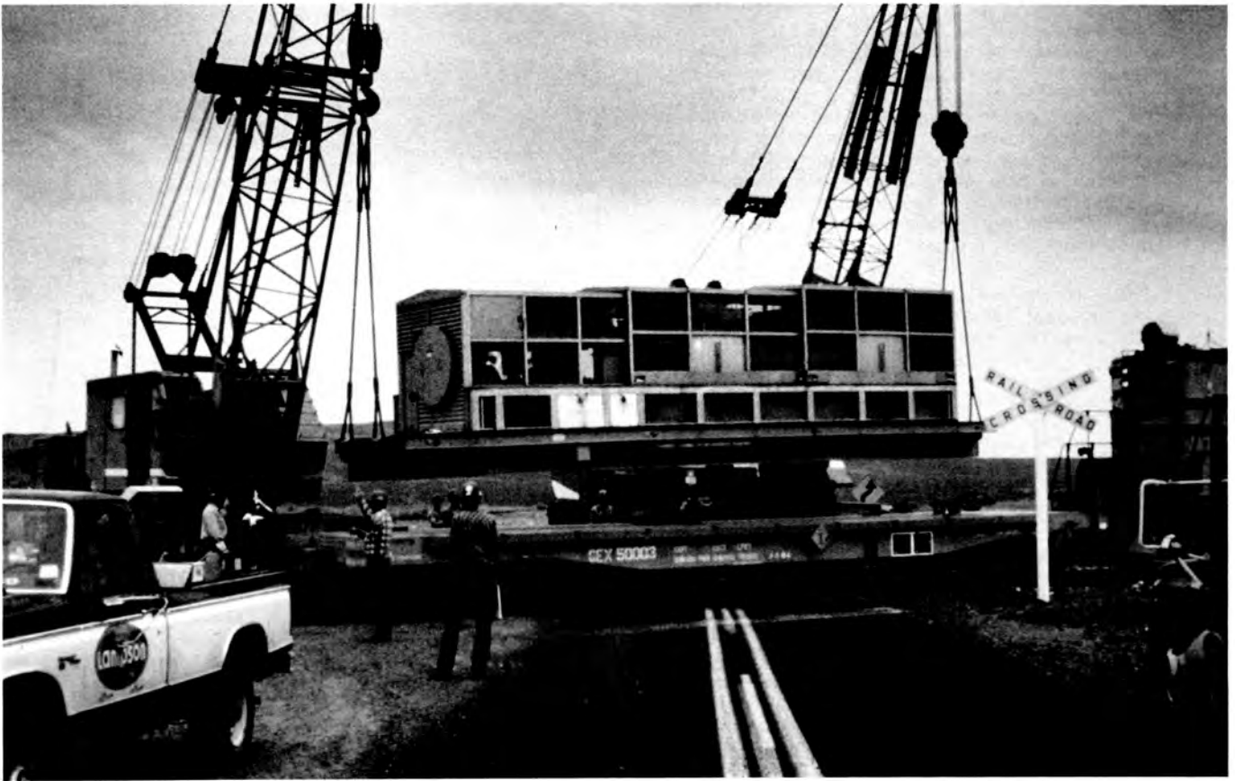
Fig. 2. Cask removal from railroad transport car.
