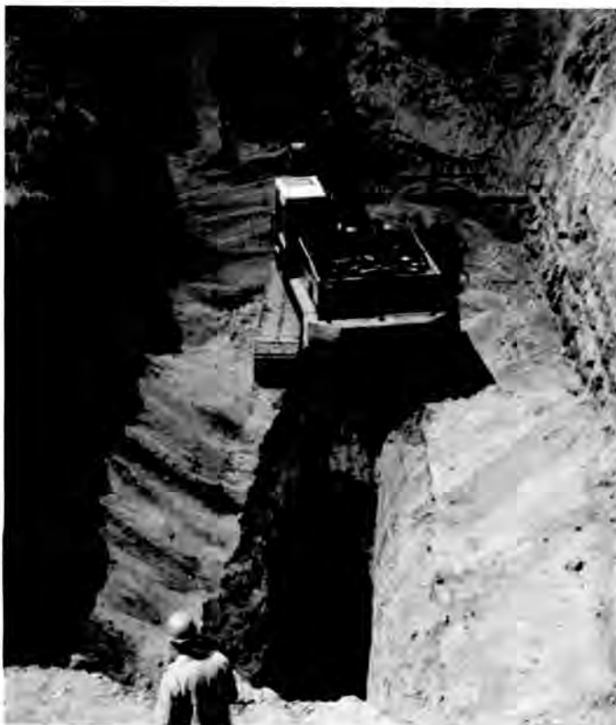
Fig. 4. Excavation of NTS Disposal trench.
