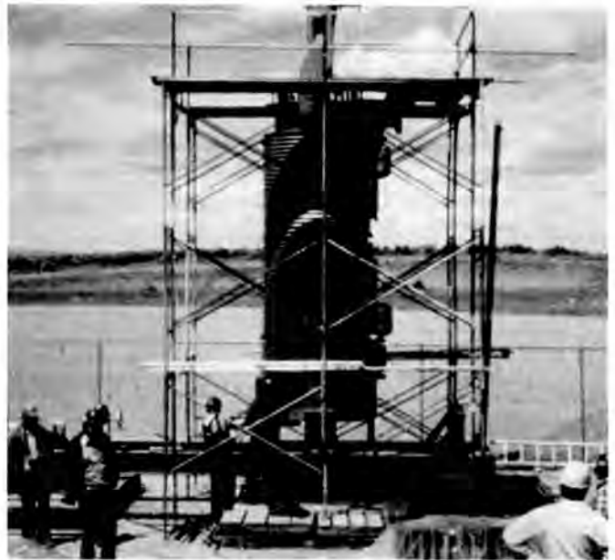
Fig. 5. IF-300 positioned vertically in cask turning fixture.
