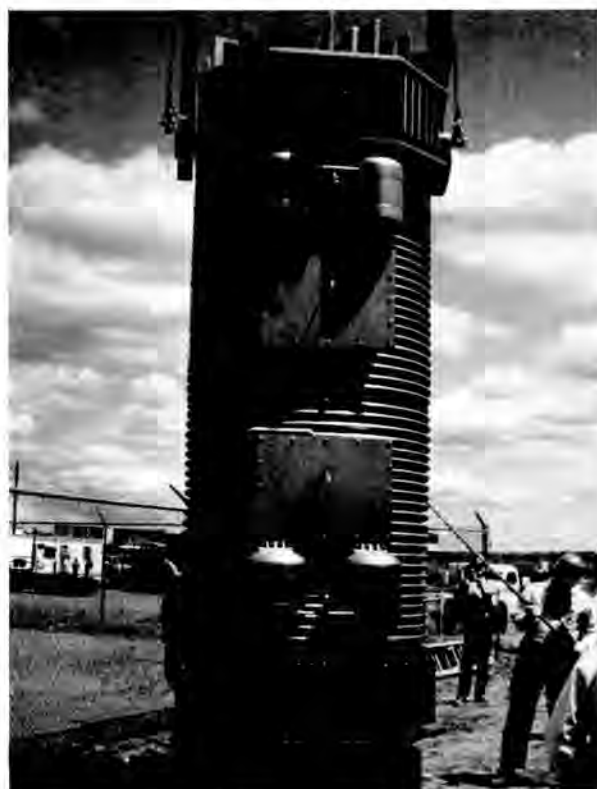
Fig. 1. General Electric IF-300 transportable cask.
