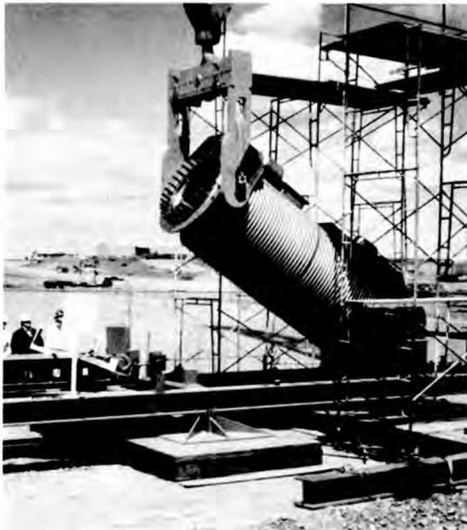
Fig. 6. Rotation of IF-300 to the horizontal off-loading position.
