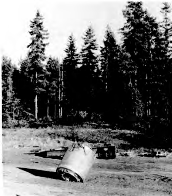
Fig. 3. Twenty-Five Foot Top Corner Drop.
