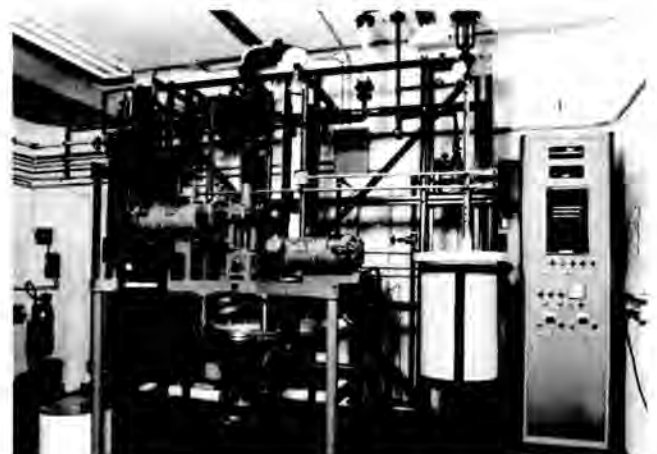
Fig. 2. AZTECH Pilot plant system.
