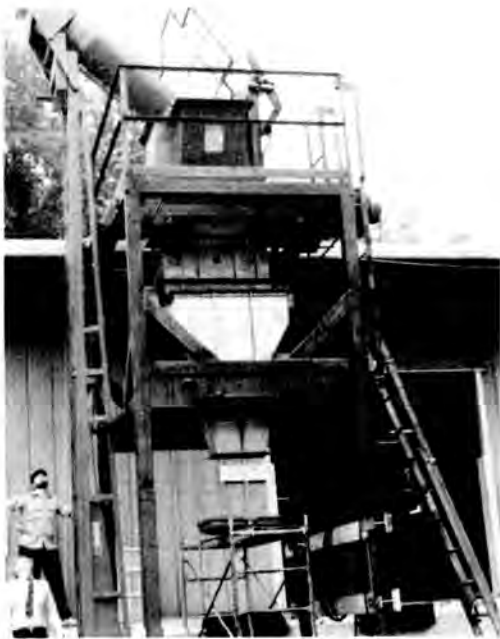
Fig. 4. Photograph of Assembled Feed Preparation System.
