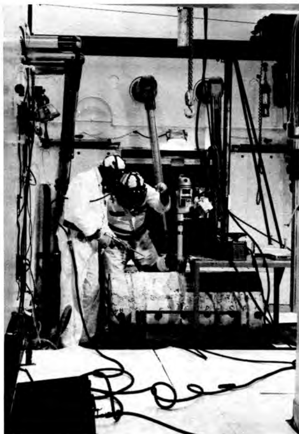
Fig. 5. Core drilling of the concrete waste form.
