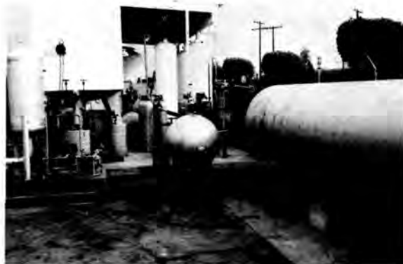
Fig. 2. test system viewed from downstream
