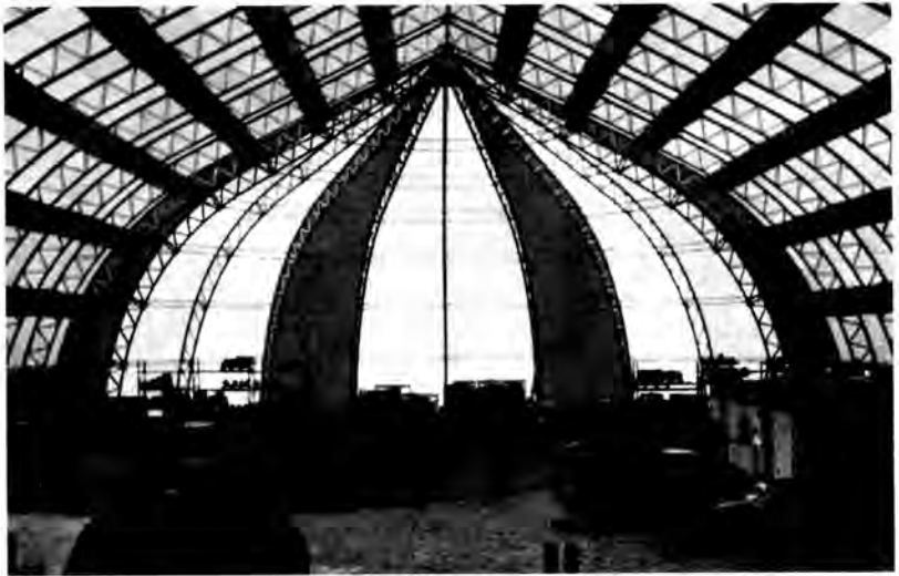
Fig. 4. Typical tension structure, 120 ft x 240 ft, general warehouse (photo courtesy of Sprung Instant Structures, Inc.).
